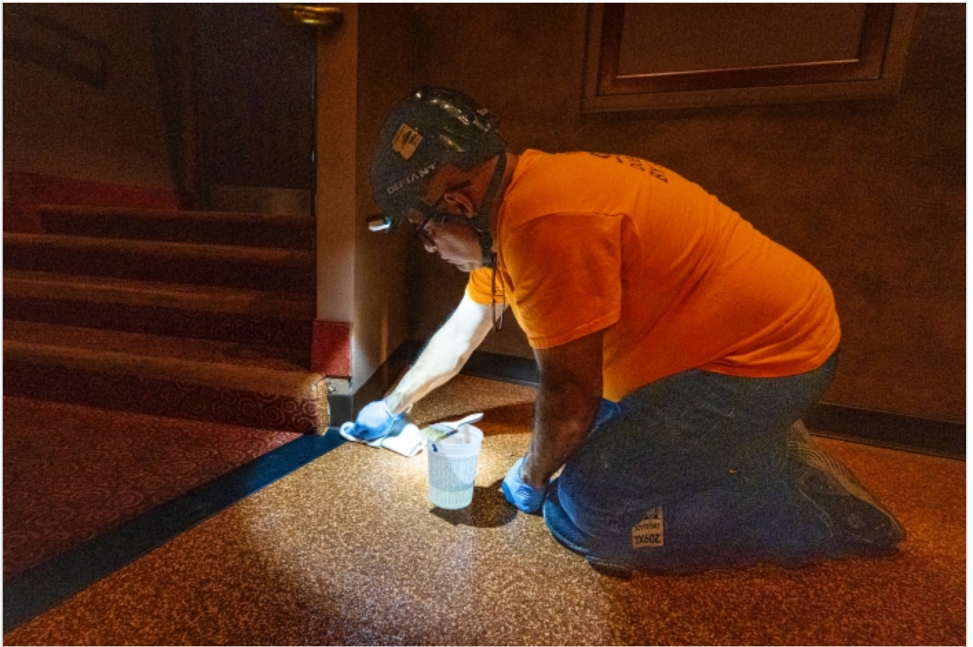
Noe Gonzalez, the site superintendent with Tempe-based Techniquex, does finishing work with the flooring sealant at ASU Gammage. Techniquex applied the new floor epoxy after workers from Mesa-based Southwest Surface Blasting stripped the floor down to the cement.
