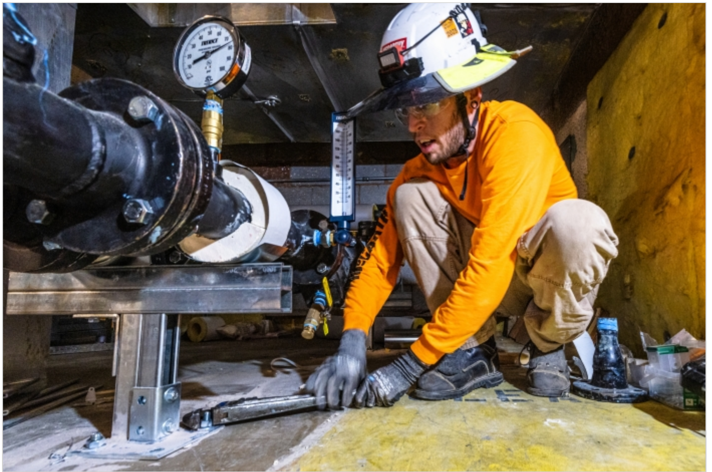
Paul Rayner, pipe fitter for McCarthy Building, tightens bolts for the new HVAC system at ASU Gammage.
