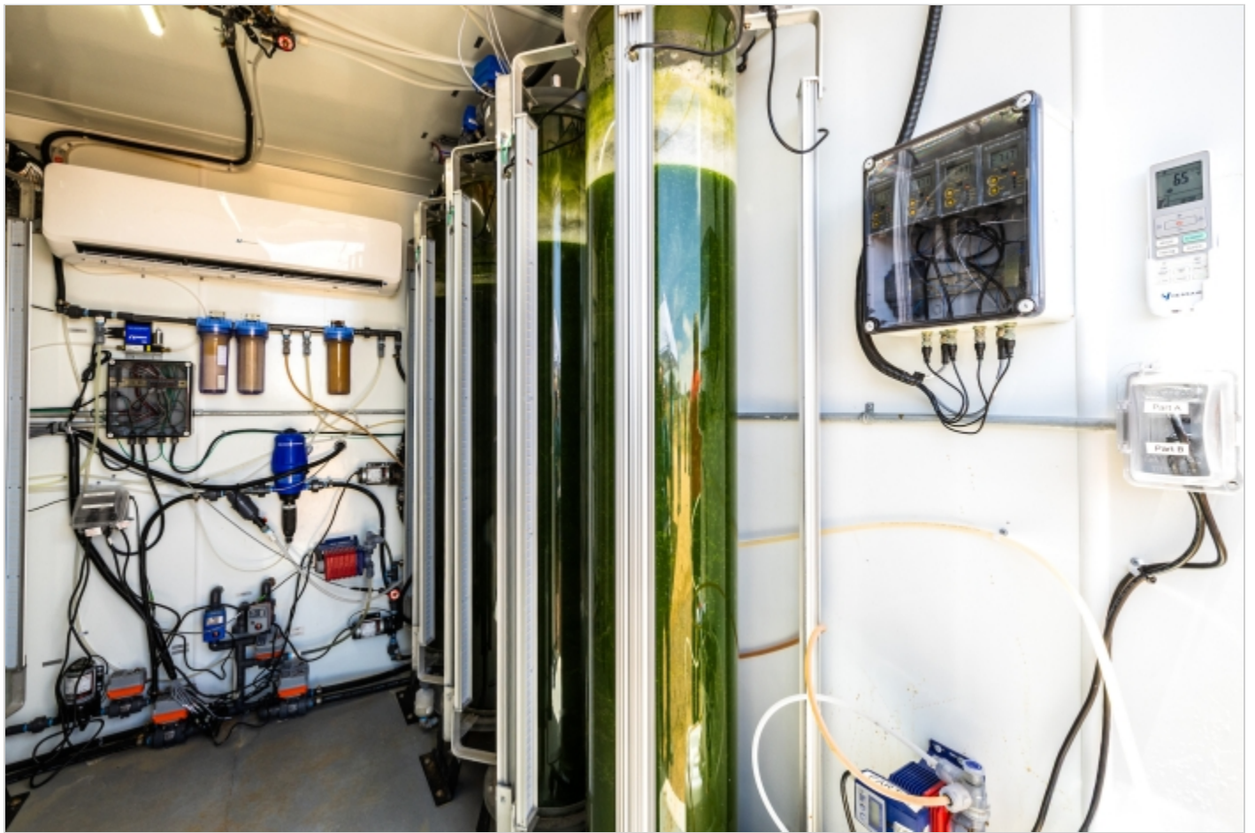
Live, native microalgae are produced onsite in algae production vessels at Curry Farms and injected directly into the irrigation system.
